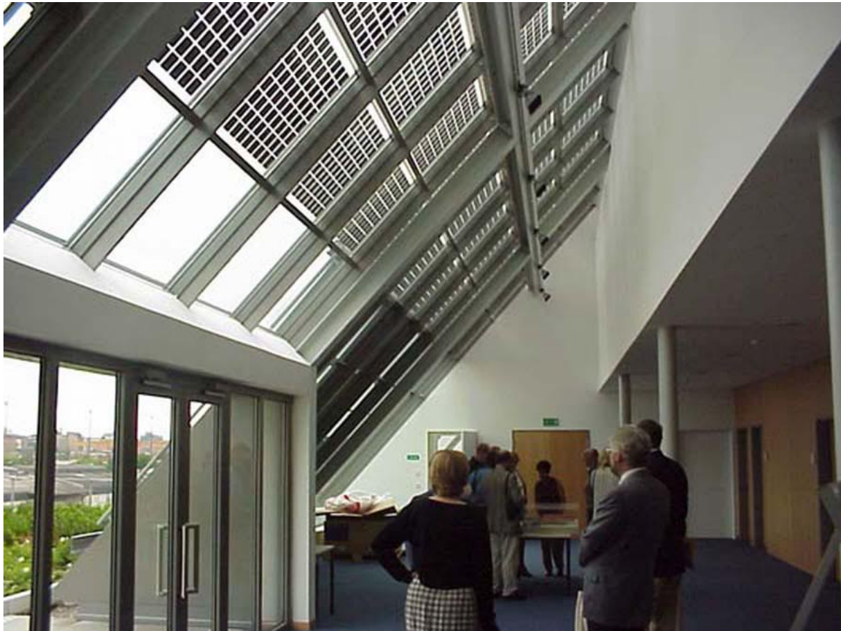
Fig. 4. An example of a façade using partially transparent photovoltaic panels, providing both PV and daylighting.
